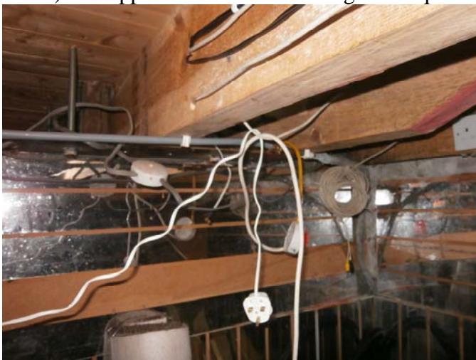
5) Unsupported cables and wiring that requires further investigation.
